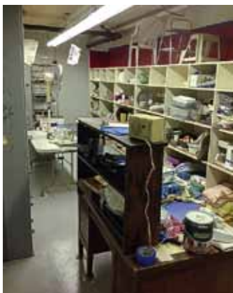
1st coat floor painted
